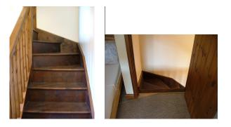
There are nine steps along dog leg staircase which lead to the Caradoc. The steps are 74cm wide. There is not a full handrail on the staircase. The bedroom door opens directly onto the staircase.
