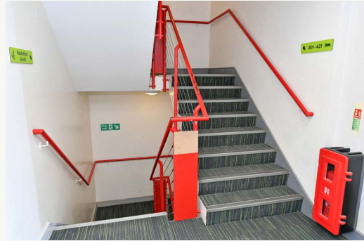
Carpeted staircases with non-slip nosing and a handrail on either side.
