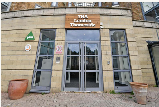
Entrance door with intercom/buzzer system.
