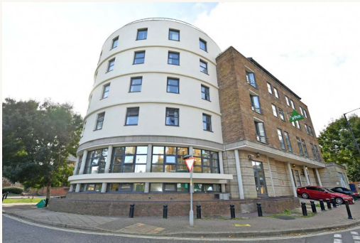
View of YHA London Thameside from Rotherhithe Street looking west.
