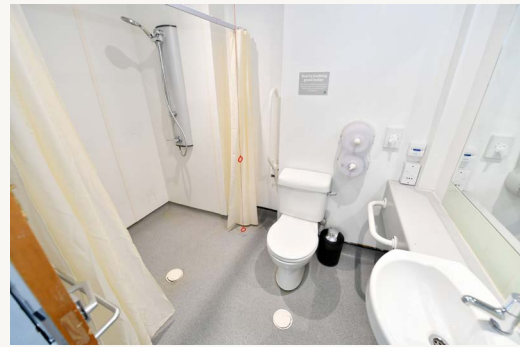
Accessible toilet and wheel-in shower.
